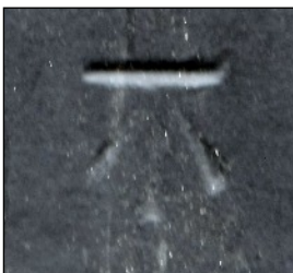
It has to be said that this benchmark has almost been obliterated by someone having painted the bottom of the building with black paint. The benchmark was noticed only because the sun was shining on it that day and cast a shadow which drew attention to the benchmark
